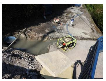
This picture, looking west towards The Chalk, shows the work in progress. The spring box is the blue drum to the left of the picture. The channel going into the stream takes the pipe to discharge the water into the nascent River Iwerne. The second box is ten metres further west.
