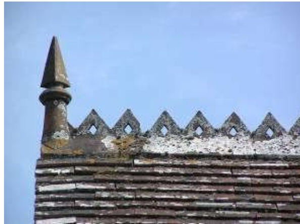
Ridge tiles and finials on Sparrow Cottage
