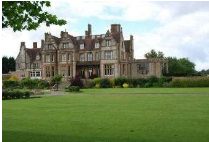
Wolverton House, now Clayesmore School
