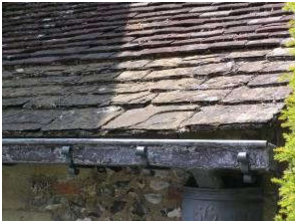
Stone tiles on the Oak House
