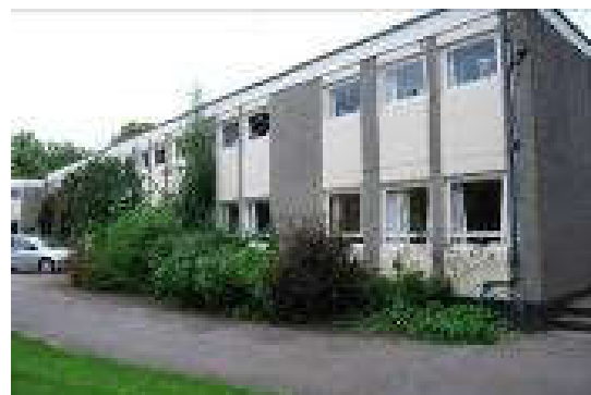
A more unsympathetic classroom block
