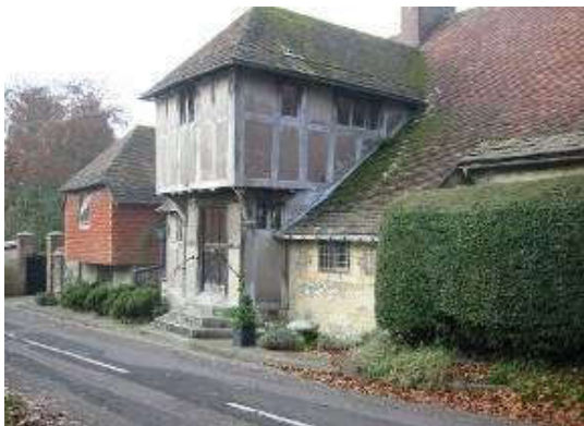
Oak House timber framing with brick nogging.
