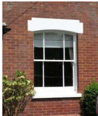
Vertical bordered sashes, Post Office Road
