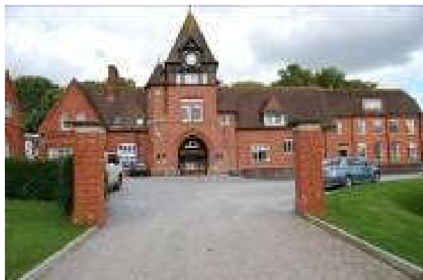
Clayesmore Stable Block
