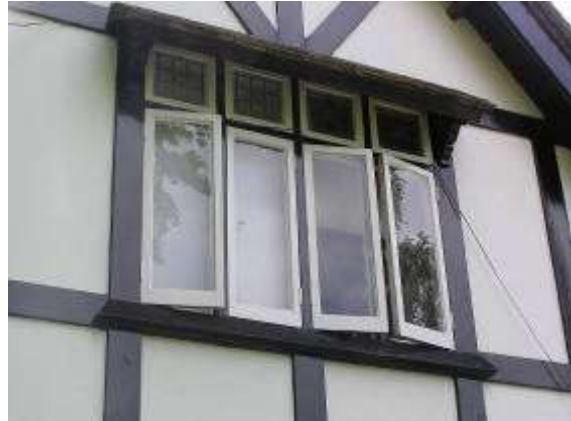
Timber casements with clerestory lights on Church Path
